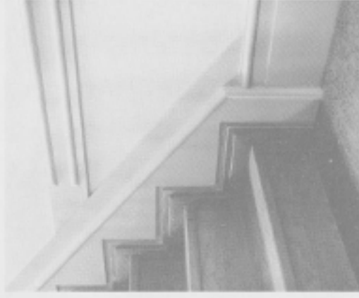
21 Details of wall treatment in No 63.
